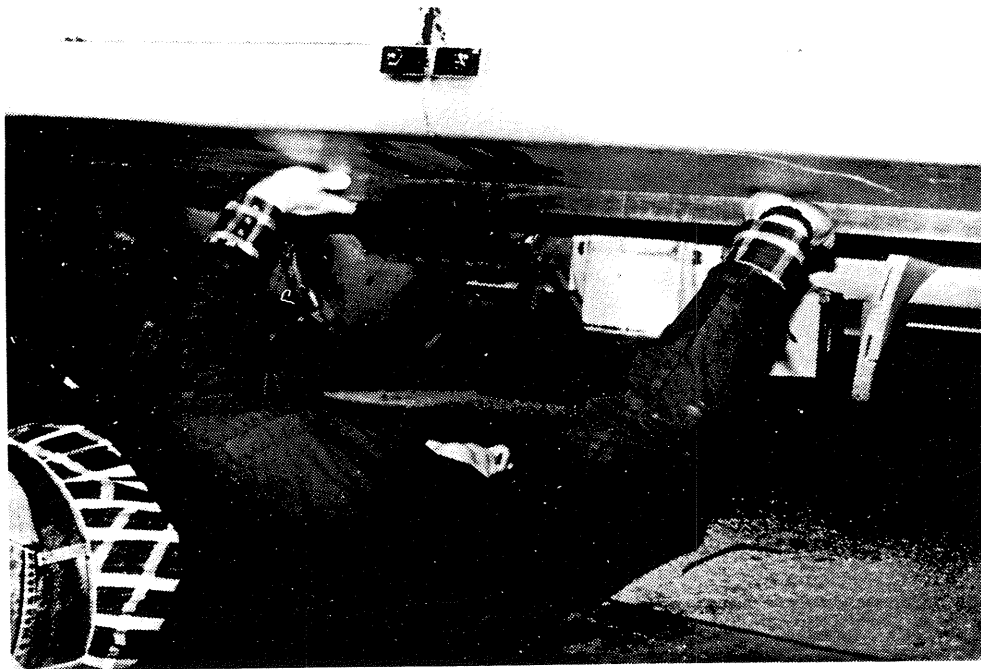
Screed Flatness Check - Straightedge Method Figure 11
