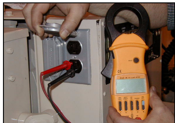
Figure 34 Setting Generator Frequency
