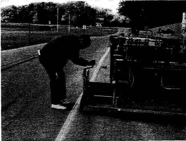
Figure 4-12 – Lowering End Gate
