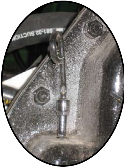
Gear Box fluid level dipstick.
