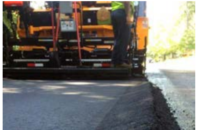
Figure 4-61. Paving with Berm Attachment
