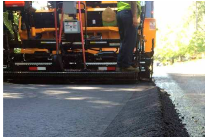
Figure 4-65. Paving with Berm Attachment
