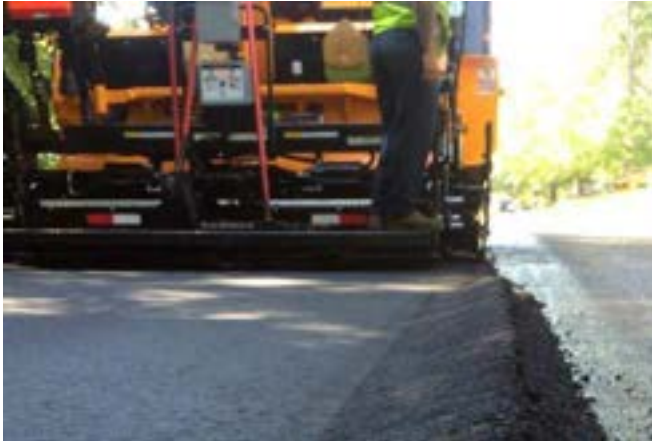
Figure 4-68. Paving with Berm Attachment
